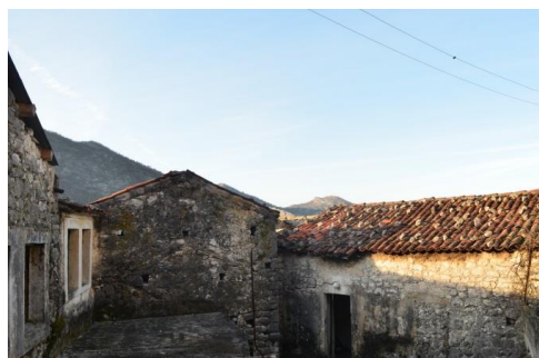
Figure 6. Roofs in village Godinje
